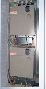
Frequency drive (system) Inverter
