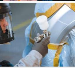
**Apply clearcoat.**Blend in clearcoat. For transitions fade out Standox Smart Blend Plus.
